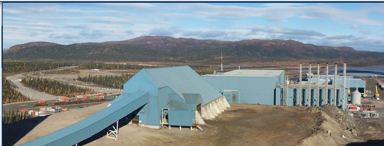
Voisey's Bay Concentrator Complex
